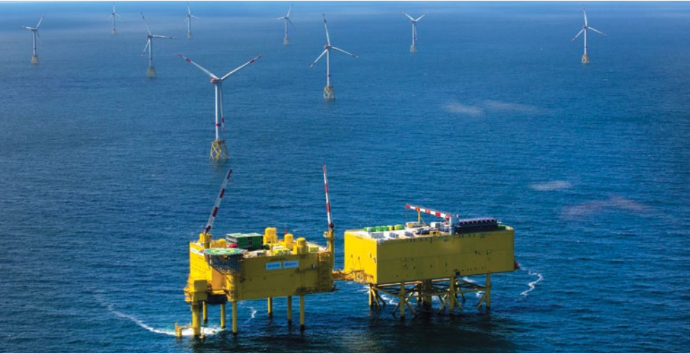
Converter substations in Germany's Nordsee OST wind farm
